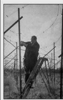
**Figure 1:** Our technician Don Rolph and the four-acre telescope. One row of antennae goes behind Don's right shoulder, and another runs from the top righthand corner of the photo. Twin-wire feeder from an antenna curves down past Don's head and joins a horizontal run of twin-wire feeder. The slanting beams carry the reflector (tilted to look at the ecliptic); the reflector is made up of wire, too fine to be seen in the photo."
