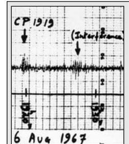
Figure 2: The first detection of the first pulsar, occupying about one-quarter inch of chart paper. About five minutes later is a short burst of low level interference. This signal has been high-pass filtered, to remove the telescope's interference pattern. (Mullard Radio Astronomy Observatory.)
